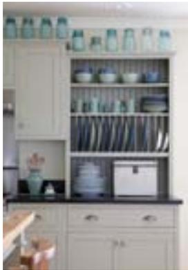
**FACE FRAME:** In this traditional-look construction, a solid-wood frame attaches to the front of the cabinet box. Hinges, hidden or visible, attach the door to the frame. Because the frame overlaps the door opening, drawers must be slightly narrower than the cabinet box. If you would like to add decorative accessories, such as corbels and fluted stiles, this option is a good choice.
